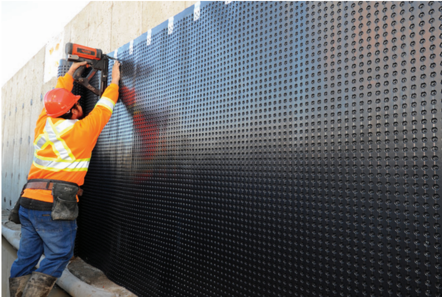
INSTALLING SPEEDCLIPS EVERY 30CM (12")
