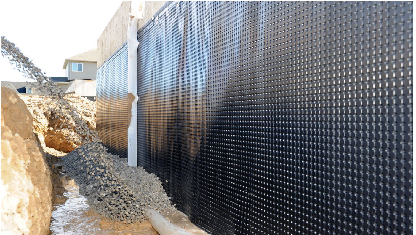
BACKFILLING OVER THE FOOTING DRAIN
